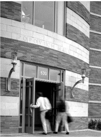
Popovich Hall, the school's new state-of-the-art graduate facility, houses classrooms, meeting rooms and the latest computer technology. This addition to the Marshall School complex opened in fall 1999.
