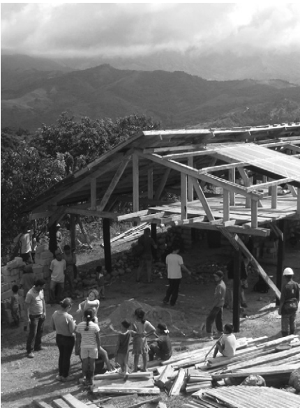
In cooperation with the Global Architecture Brigades, School of Architecture students construct a multipurpose building for a Panama community farm recently devastated by fierce winds. The students' innovative design diverts winds and ensures stability.
